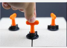
Hold the handle and keep it unmoved to tighten the nut to reach a fixed leveling
